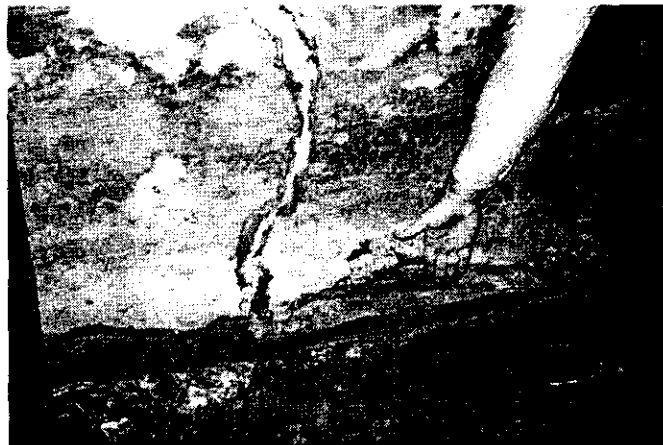
Earthquake? Blasting damage in Western Pennsylvania ascribed by OSM to unrecorded seismic events.
