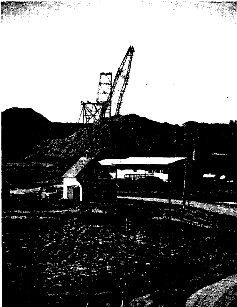
Howdy, Neighbor. “Dragline” looming over North Dakota farmhouse.
