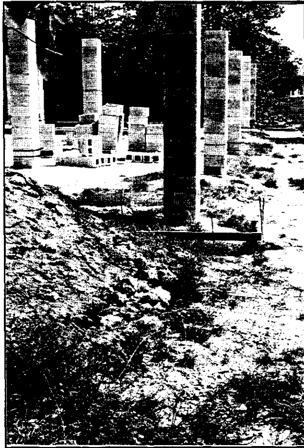
THE CORPS IN INACTION. Illegal “dream house” being built in wetlands.
