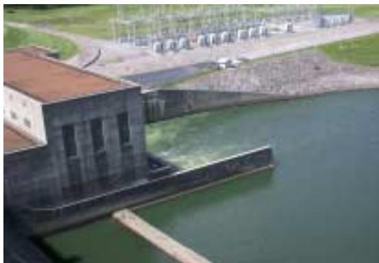
Center Hill Dam power generation facility
