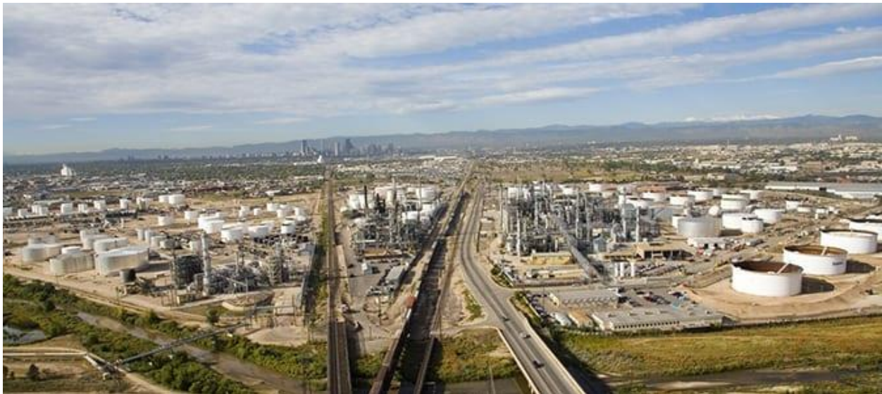
Suncor Refinery, Image at suncor.com
