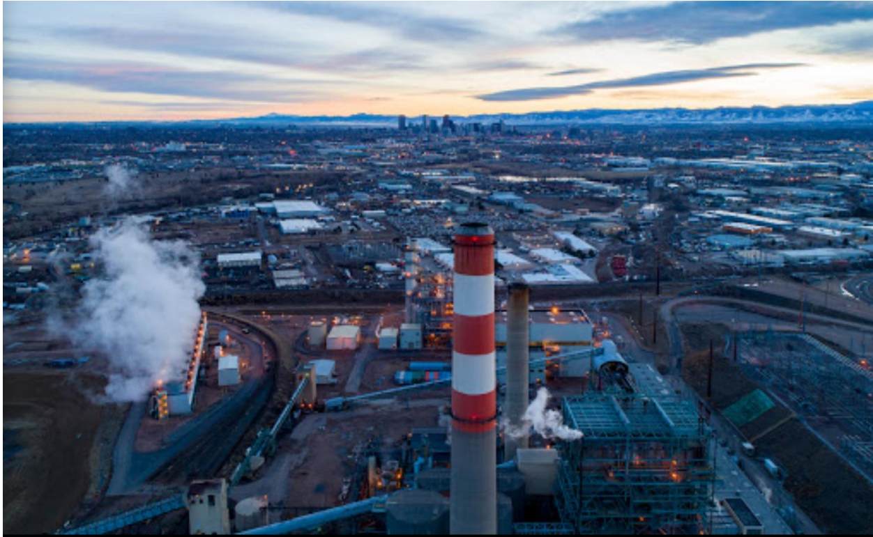
Cherokee Power Plant, photo by Gregor Tokarski 1/19
