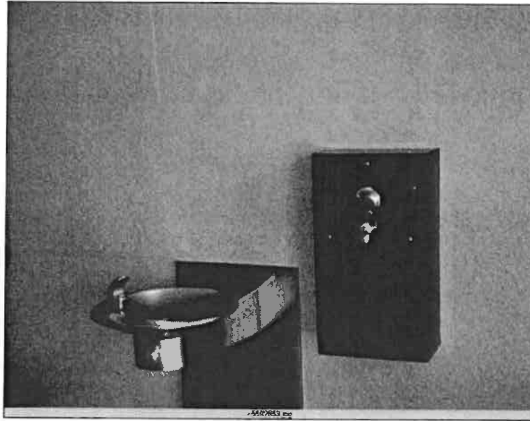
A newly installed water bottle filler at the Tucson Mountain District's Red Hills Visitor Center. Visitors were using the device before the installation crew had left the site!
